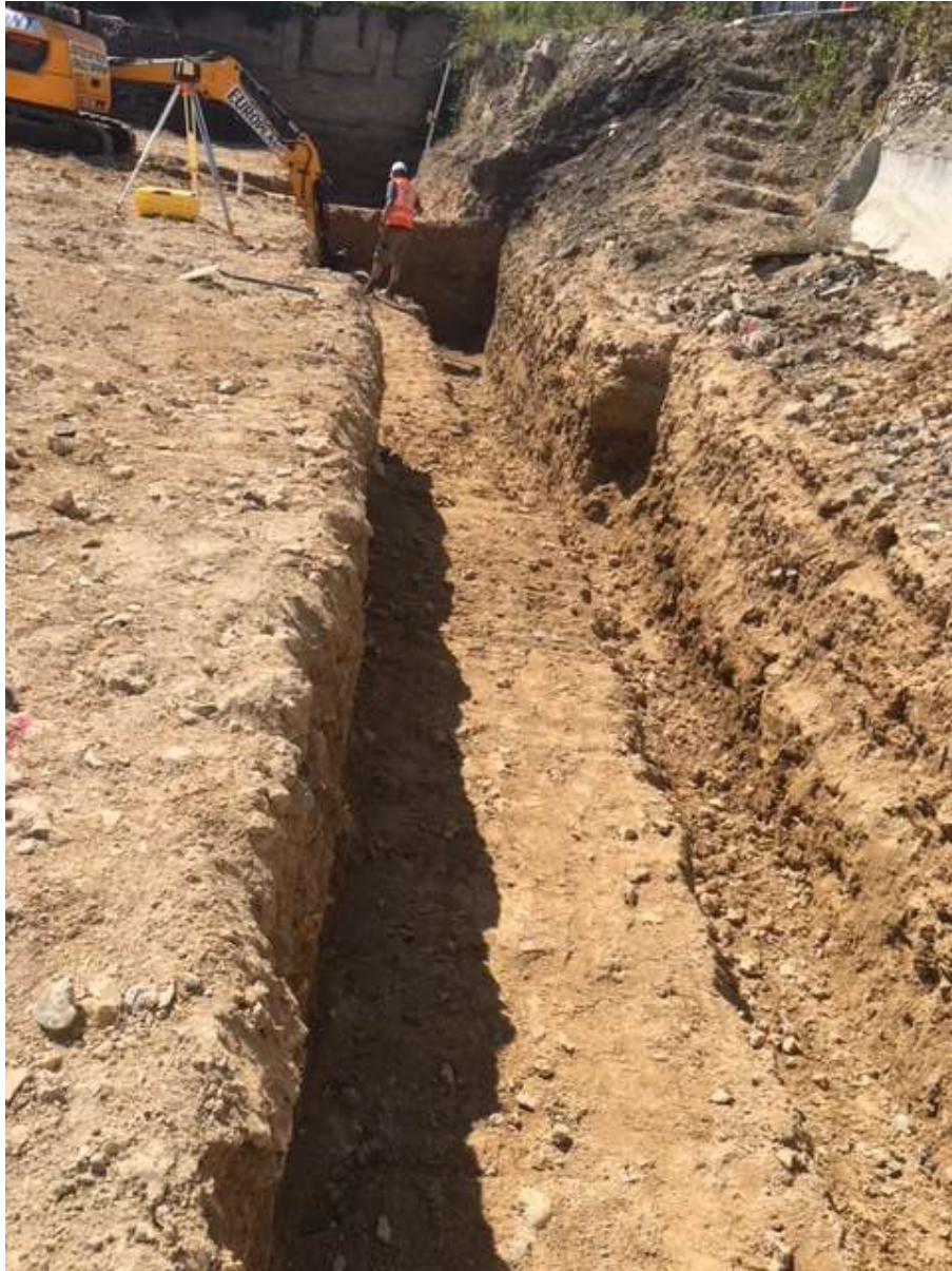
Plate 7. View of trenches (looking W)
