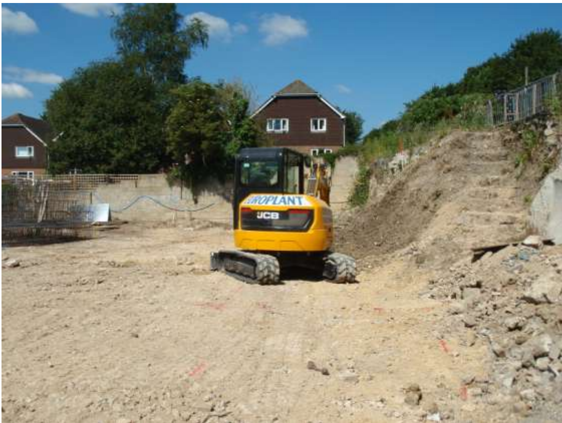
Plate 3. View of ground reduction (looking W)
