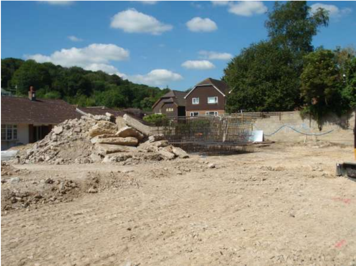
Plate 4. View of site clearance (looking SW)
